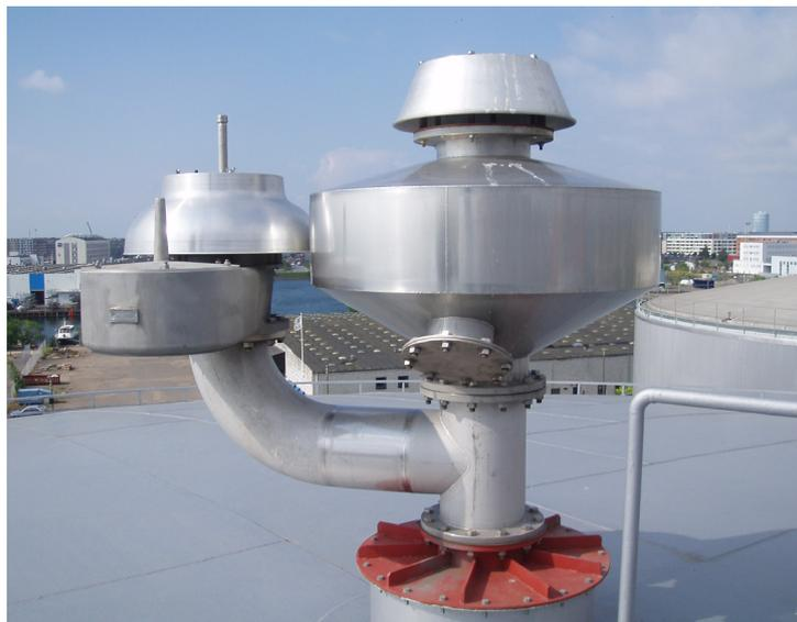
*Standard Tank Vent Odour Filter in a selfcontained version, with a breather valve (pressure/vacuum) regulation, for smaller tanks.*
